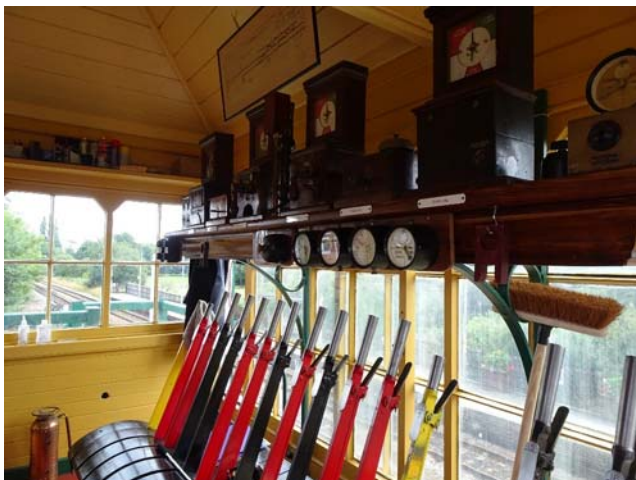
Lowdham Signal Box
