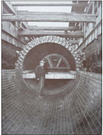
Construction of a sewer main, c1890
