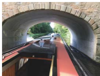
Rebuilt bridge at Elland
