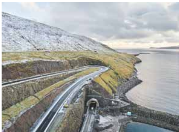
The 10-8 km long Sandoy Tunnel connecting the main island of Streymoy with Sandoy to the south opened on 21 December 2023.
