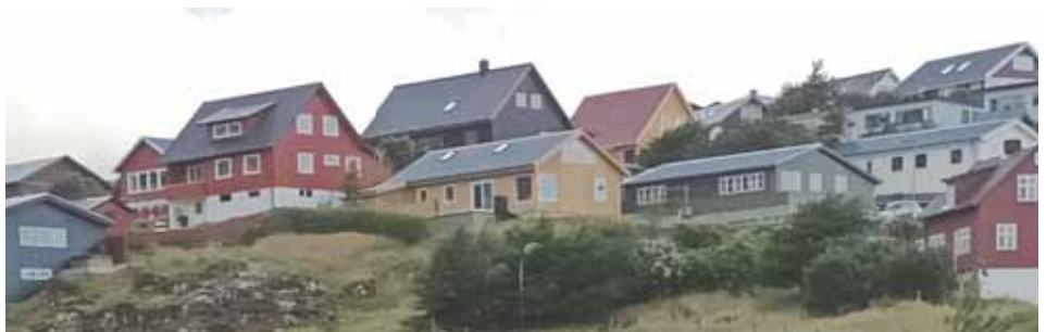
Many grey corrugated steel roofed buildings
