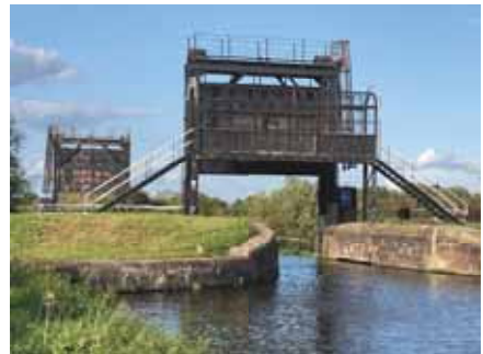
The impressive guillotine gates over the River Don which are closed to prevent the canal being overwhelmed when the river is in flood
