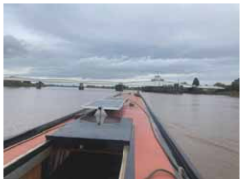
Approaching Goole railway swing bridge
