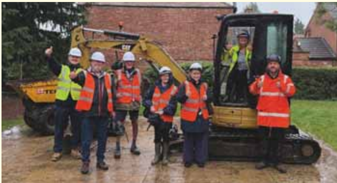
Work Starts on the Community Garden
