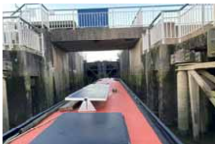
Barmby Barrage and the bridge
